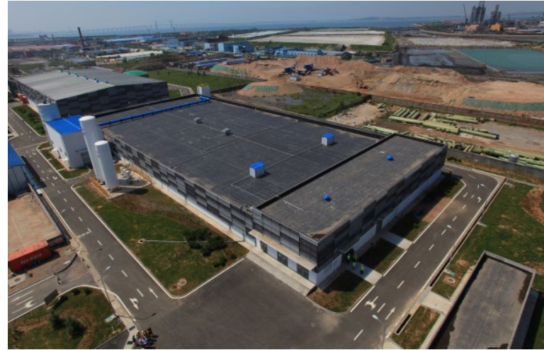
Qingdao SWRO Desalination Plant, Qingdao, China
